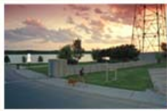
FLOOD DAMAGE REDUCTION
